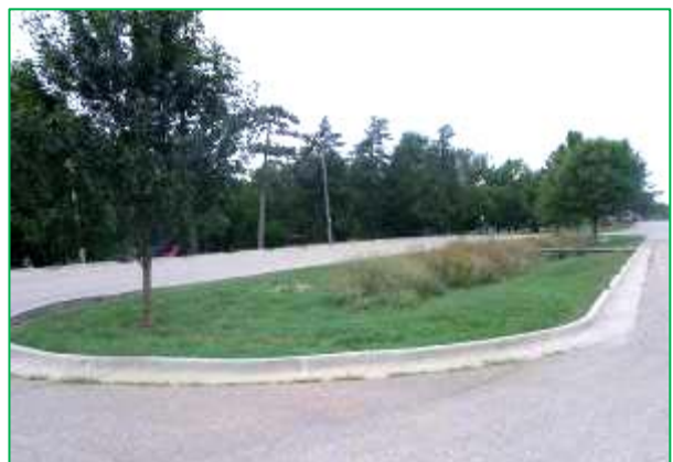
Above left: An example of an existing grassed channel in Downtown Topeka at SW 8 th and Jackson Street. Above right: An existing bioswale within the Hillcrest Community Center parking lot used for storm water management.
