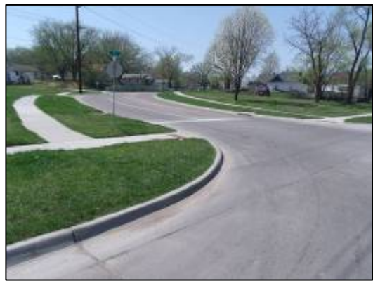
Above left: foot bridge constructed by the homeowner to access the street and the mailbox from the front of the house due to missing infrastructure. Above right: re-built curbs and gutters, and new sidewalks constructed at the intersection of SE 6 th and 10 th Avenue in the East Topeka neighborhood.
